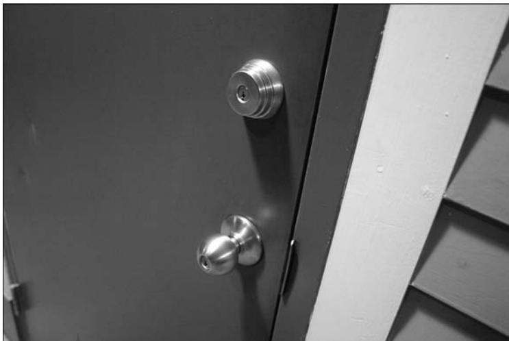
Figure 6.4 Serrures cylindriques.
